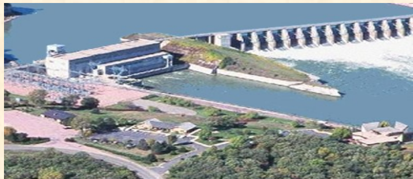
Gavins Point Dam
