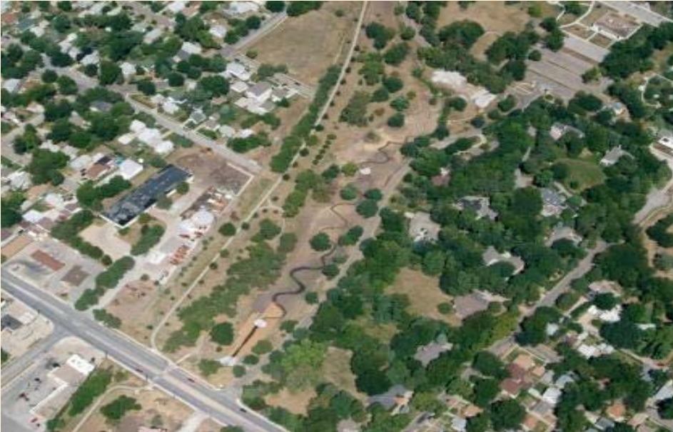
Meandering Channel North of South Street
